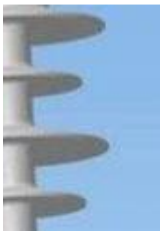
Figure 4 – Example of alternate rib length on the polymer insulator
