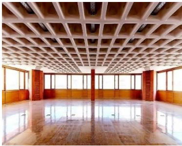
Figure 1, Bottom view of Waffle slab (19)
