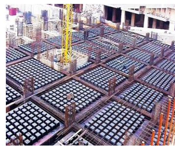
Figure 3, Waffle slab's Formwork (21)
