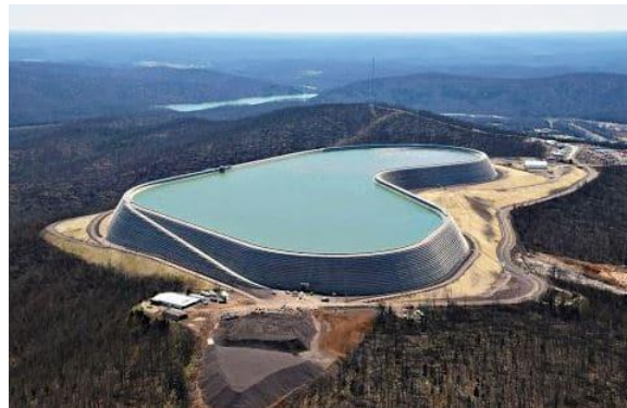
Fig. 10. Taum Sauk Dam Constructed Using Roller Compacted Concrete
