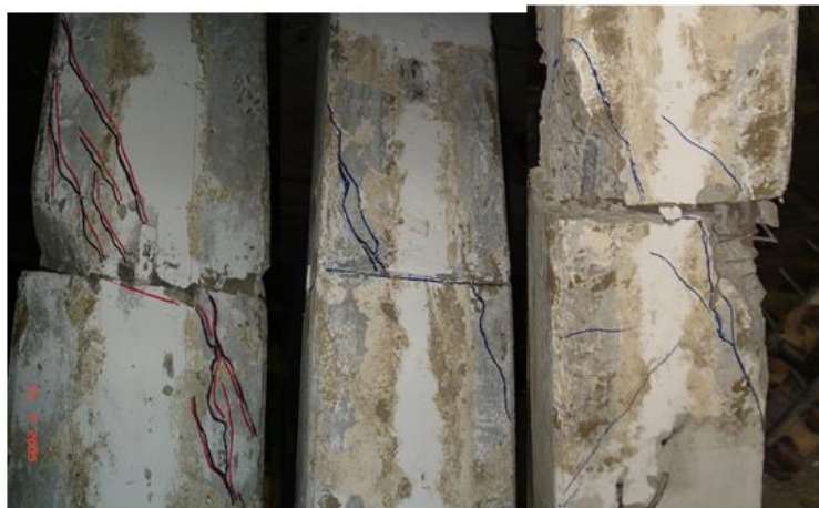
Fig. 11. Type of destroyed samples after testing
